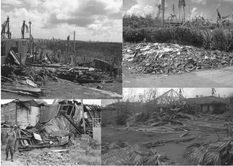
4.2. Photographs showing damage caused by Hurricane Ike in 2008, taken by the author and colleagues. Clockwise from bottom-left: two different modern house designs destroyed by the hurricane, unusable broken house tiles collected for disposal following the hurricane, and one Precolumbian house from the “Taino” heritage village of El Chorro de Maita being rebuilt six days after the hurricane. Photos by (clockwise from bottom-left) Roberto Valcárcel Rojas, Roberto Valcárcel Rojas, and Jago Sheets.
