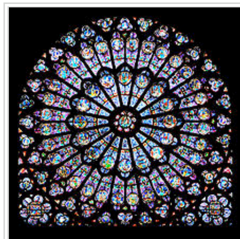
Gothic stained glass rose window of Notre-Dame de Paris. The colors were achieved by colloids of gold nano-particles.
