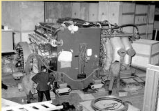
Installing the Heavy Liquid Bubble Chamber.
