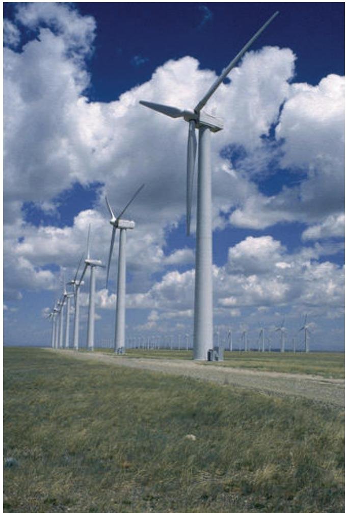
Wind power is a primary renewable energy source. Wind turbines are operated across a range of wind speeds. For a majority of the time, wind turbines operate below the rated wind speed; the so-called Region-2 operation. The primary objective of Region-2 wind turbine control is to maximize the power output by adjusting generator torque and/or blade pitch angle.
