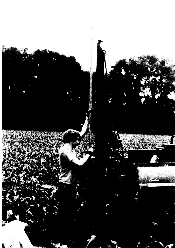
Figure 3. A mechanical coring device, called a Giddings soil sampling machine, with a coring tube attachment (owned by Dr. R. Ruhe, Indiana University).
