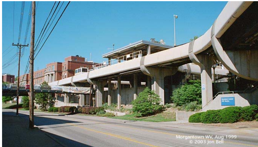
Figure 2.1 Photos of Morgantown PRT System
