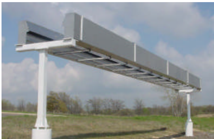
First full-scale, MicroRail guideway section
