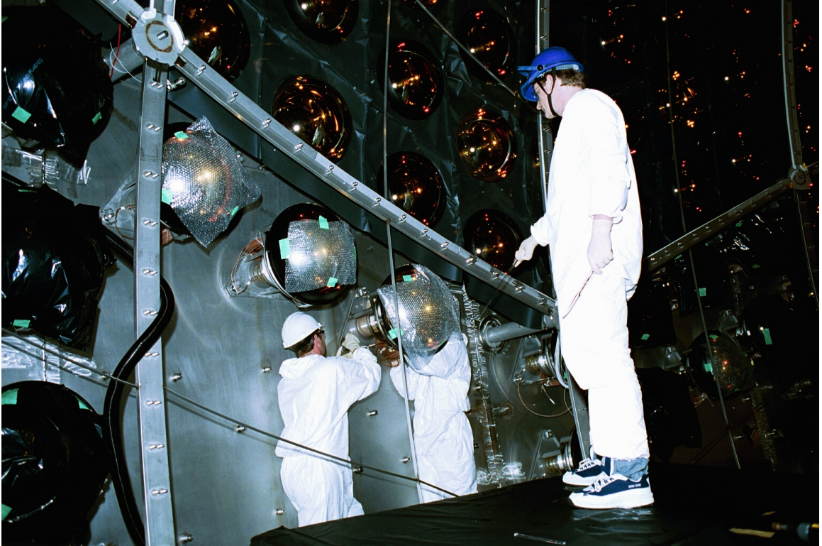
Figure 3.2: A photograph of PMT installation. The workers are, from left to right, K. McKinny (University of Alabama), the author, and J. Ritter (California Institute of Technology). Photo taken by T. Takayama (Tohoku University).
