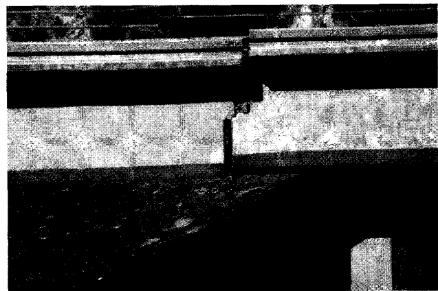
FIG. 1. In-Span Hinge on Verge of Collapse (1994 Northridge Earthquake)
