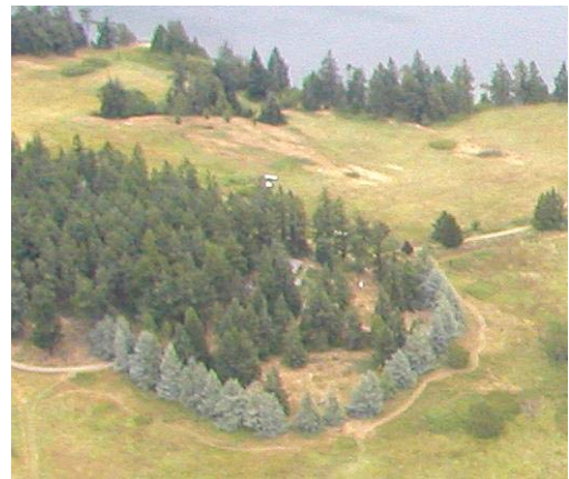
Figure 29. Oblique aerial photo showing caretakers house and partial ring of Atlas cedars. Photograph by Ken Sebens, July 2006.
