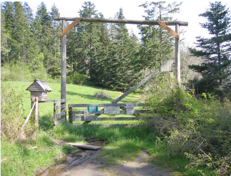
Figure 19. Public entrance at the southwest corner of Cedar Rock Preserve for day use, including parking for one or two cars and small “house” containing the visitor book. Photograph by Claudia Mills, April 2007.
