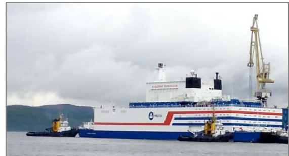
Figure 13. The first SMR on a Russian barge being towed to a Siberian coastal site.
