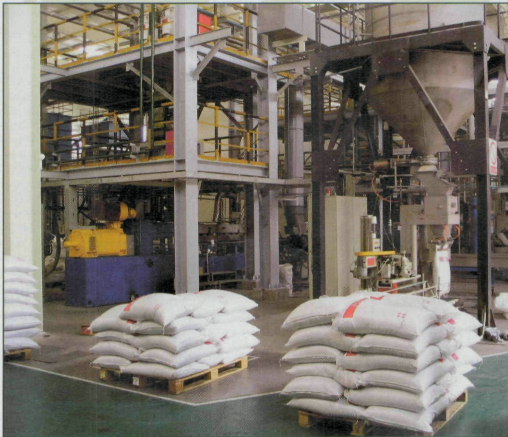
Automatic sorting at MBA's China plant produces consistent grades of ABS, HIPS, and PP from low-FR e-plastics gathered from around the world.
