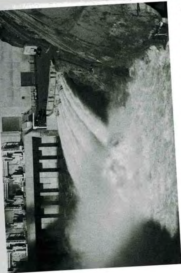
Figure 2.4 An artificial flood in progress. Water is being released at a high rate from the Glen Canyon Dam in an attempt to provide additional sandbars for river boaters in Grand Canyon. Predictive models of the sandbar configuration that resulted from the water release were unsuccessful. Photo courtesy of the U. S. Geological Survey.
