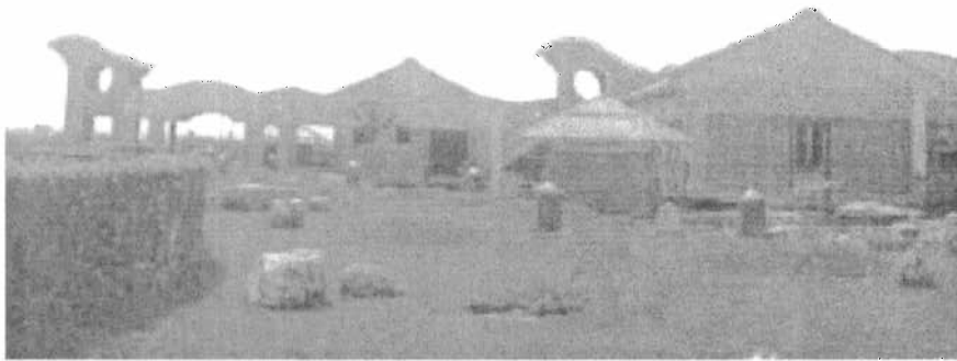
Fig. 3. Minnan-style Roof Garden, the Ilan County Hall
