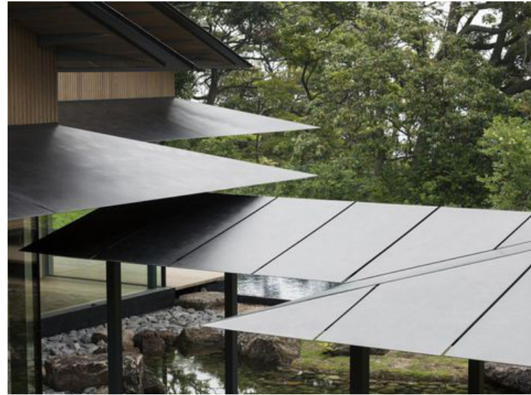
STEEL PLATE ROOF
