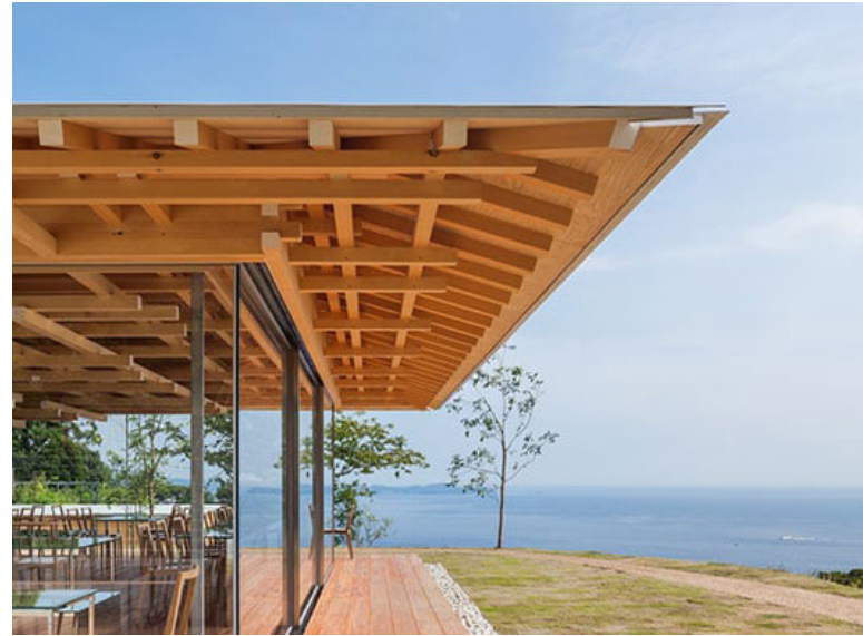
WARM WOOD UNDERSIDE
