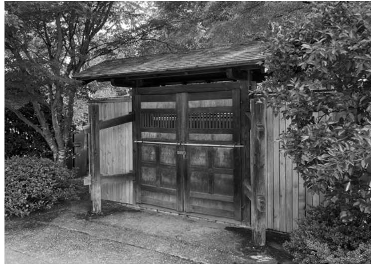
Original Entry Gate
