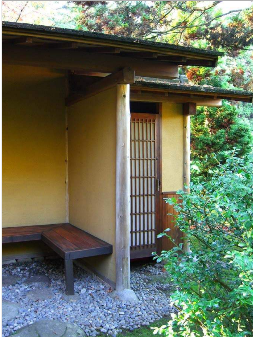
Northern end of machiai east elevation
