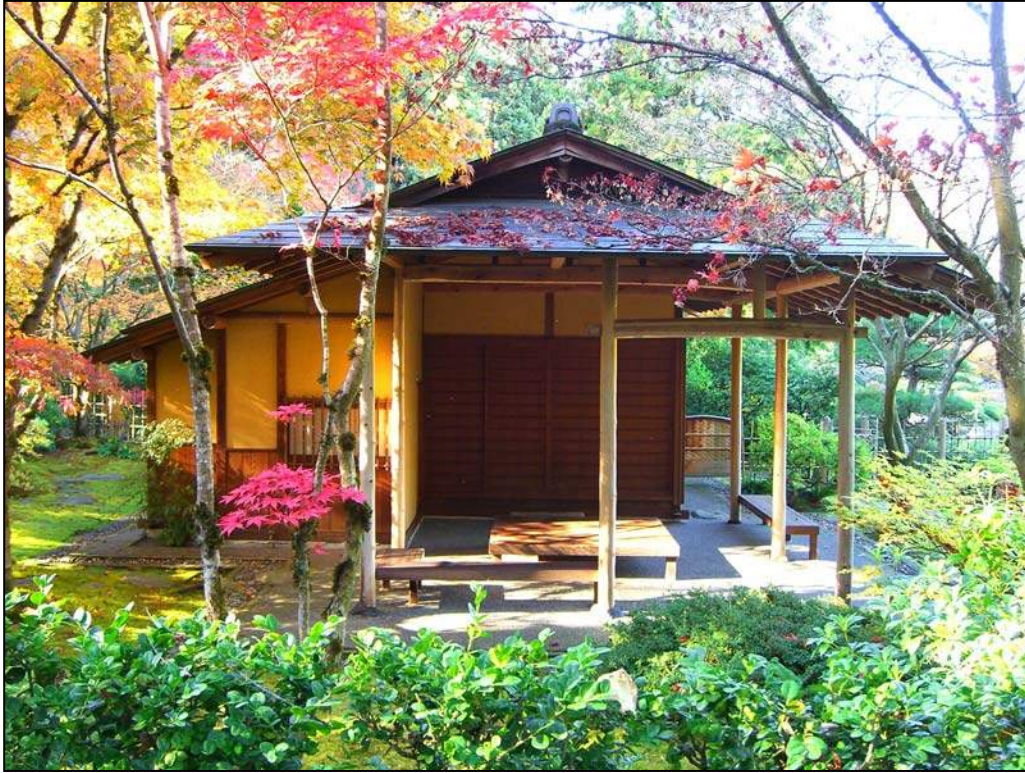
South elevation of Shoseian, Arbor of the Murmuring Pines
