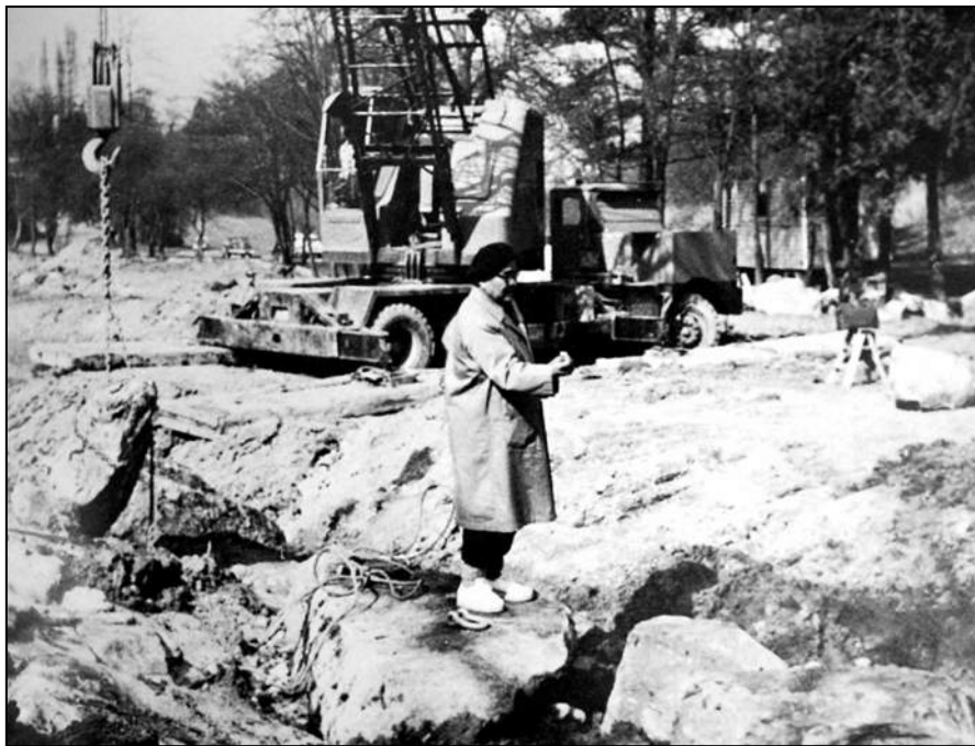
Japanese Garden under construction with Mr. Juki Iida, landscape architect, May 1960
