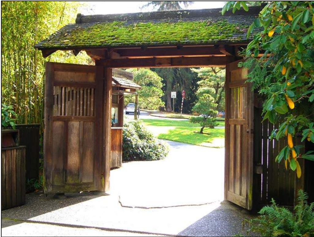
Interior View, South Entry Gate
