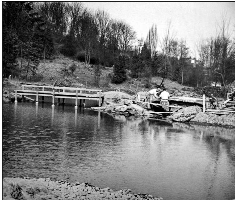
Construction of the two bridges, April 5, 1960
