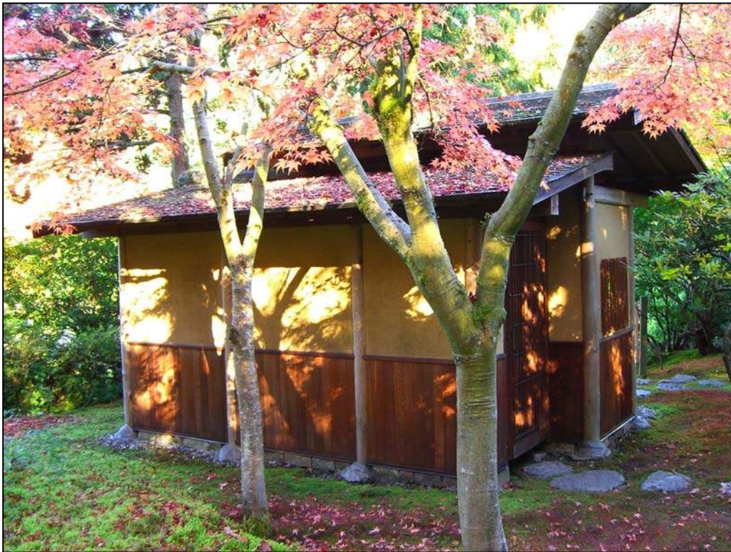
Rear west and south elevations of machiai
