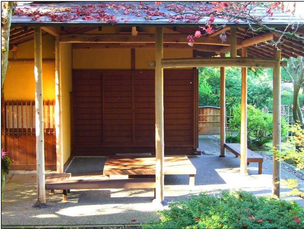
Detail of south elevation of Shoseian, Arbor of the Murmuring Pines, showing doma or covered terrace
