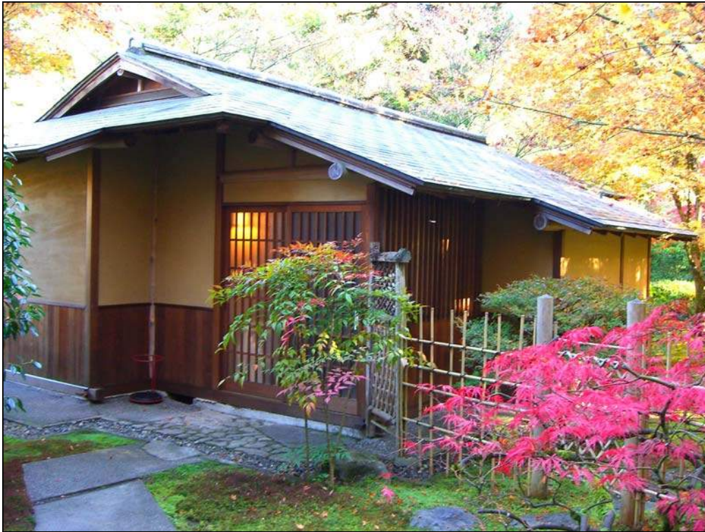
North and west elevations of Shoseian, Arbor of the Murmuring Pines
