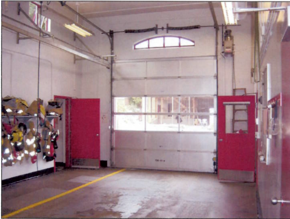
Above, view of Apparatus Room looking east. Note the clerestory windows at upper right and the arched transom over the door. The overhead door dates from ca. 1987.
