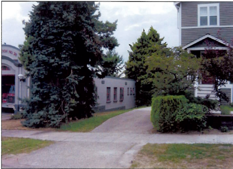
Above, view looking west, showing partial east and north facades.
