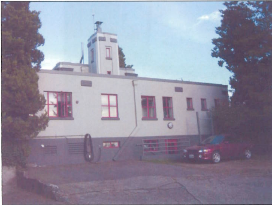
Above, partial view of the west facade looking east from alley. The parking lot is shown in the forefront, and the stair to the Basement is near the center of the facade.
