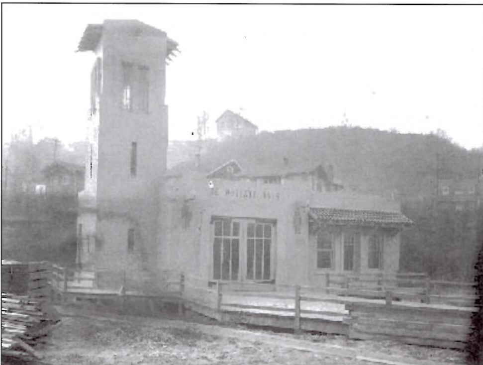
Below, view of West Seattle's Engine House Station No. 36, which was built 1918. It was the city's smallest station at that time, and the first that used the popular Spanish/Mission Revival style. Source: Seattle Municipal Archives, Item No. 2688.
