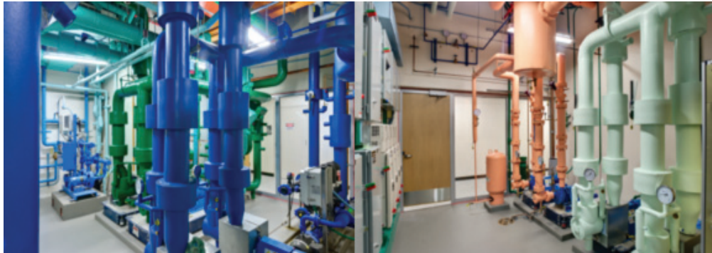
Mechanical equipment, pumps, piping, and sensors are part of the building HVAC systems.
