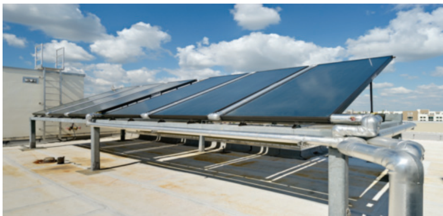
Solar photovoltaic cells on a building roof for power generation.
