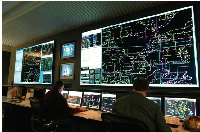
*With advanced visualization tools, power system operators can be better aware of current operating conditions and prepared to take decisive actions needed to avoid blackouts. The tools are also useful in power system planning, policy analysis, and education of the next generation of electric power engineers.*
