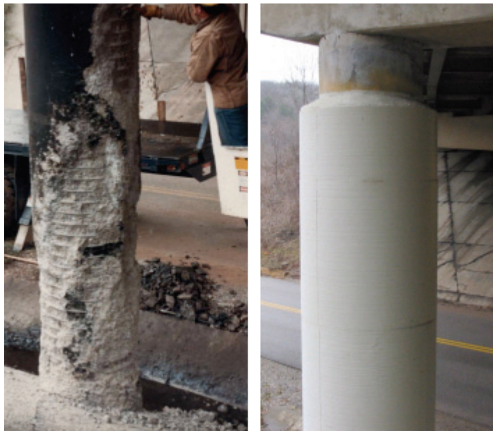
Before and after composite wrapping.
