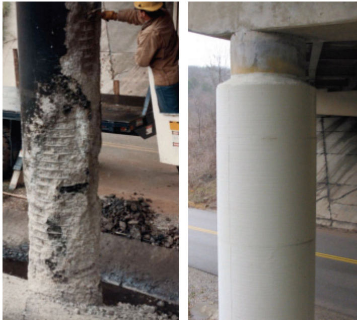
Before and after composite wrapping.
