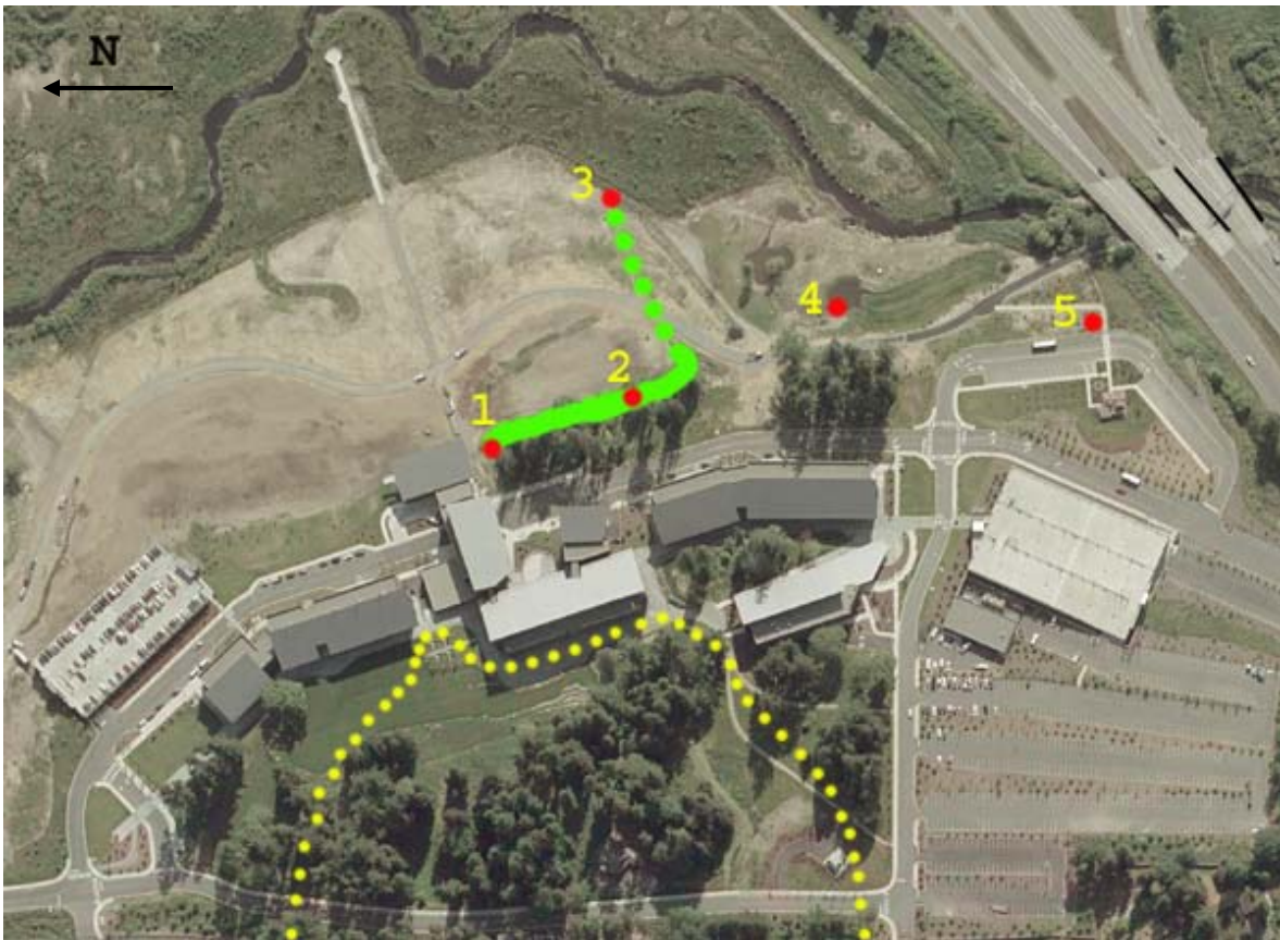
Figure 1. 2002 aerial photograph of the UWB and Cascadia Community College campus and wetland showing the location of the sampling sites. A pipe discharges groundwater at Site 1 (see Fig. 2) into a bioswale (green line). The water flows to Site 2, turns a corner and enters another pipe (see Figures 3 and 4), which extends under the wetland fringe. The pipe reemerges at Site 3, where the water is discharged into a bog before continuing as surface flow to North Creek. The dotted yellow line is a very rough approximation of the area that could contribute recharge to the groundwater that is collected in a french drain and piped to Site 1. Samples were also analyzed from a pond (Site 4) and a stormwater catch basin (Site 5). The photo is a section of a USGS (2003) high resolution orthoimage.
