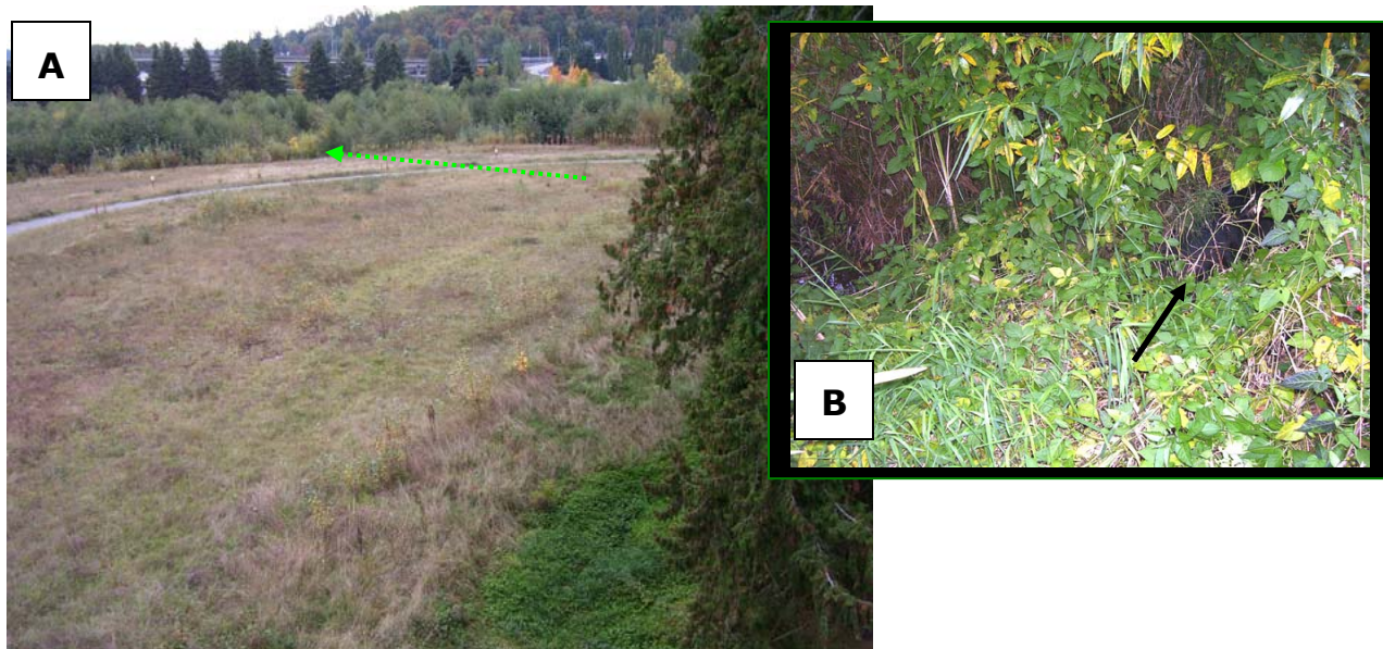
Figure 4. Photographs showing the location of Site 3. The dashed green arrow in Photo A indicates the location of the underground pipe and the discharge point at Site 3. Photo B shows the open pipe at Site 3 (black arrow) and the wet area to the left. Note the lush green growth in the bioswale (lower right of Photo A) relative to the adjacent grassy area. Photos taken on 10/9/2007.
