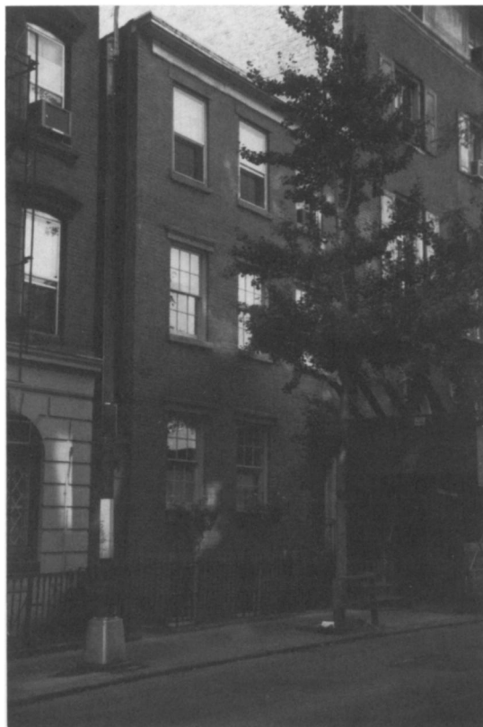
FIGURE 2. 25 Barrow Street, New York City. The sloping roof and dormer windows of this late Federal-style house were removed when the full third story was added in the 1870s.
