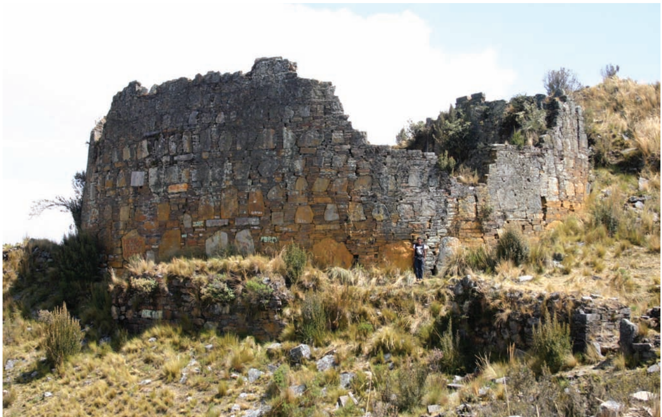
Figure 7. Circular compound c50, view from southeast. These windowless residential complexes featured an outer ring of rooms rising multiple stories and a central courtyard. The interiors appear to have been the foci of social life for different Recuay groups. Note the platform at the base of the building, and also the gateway at the lower right.
