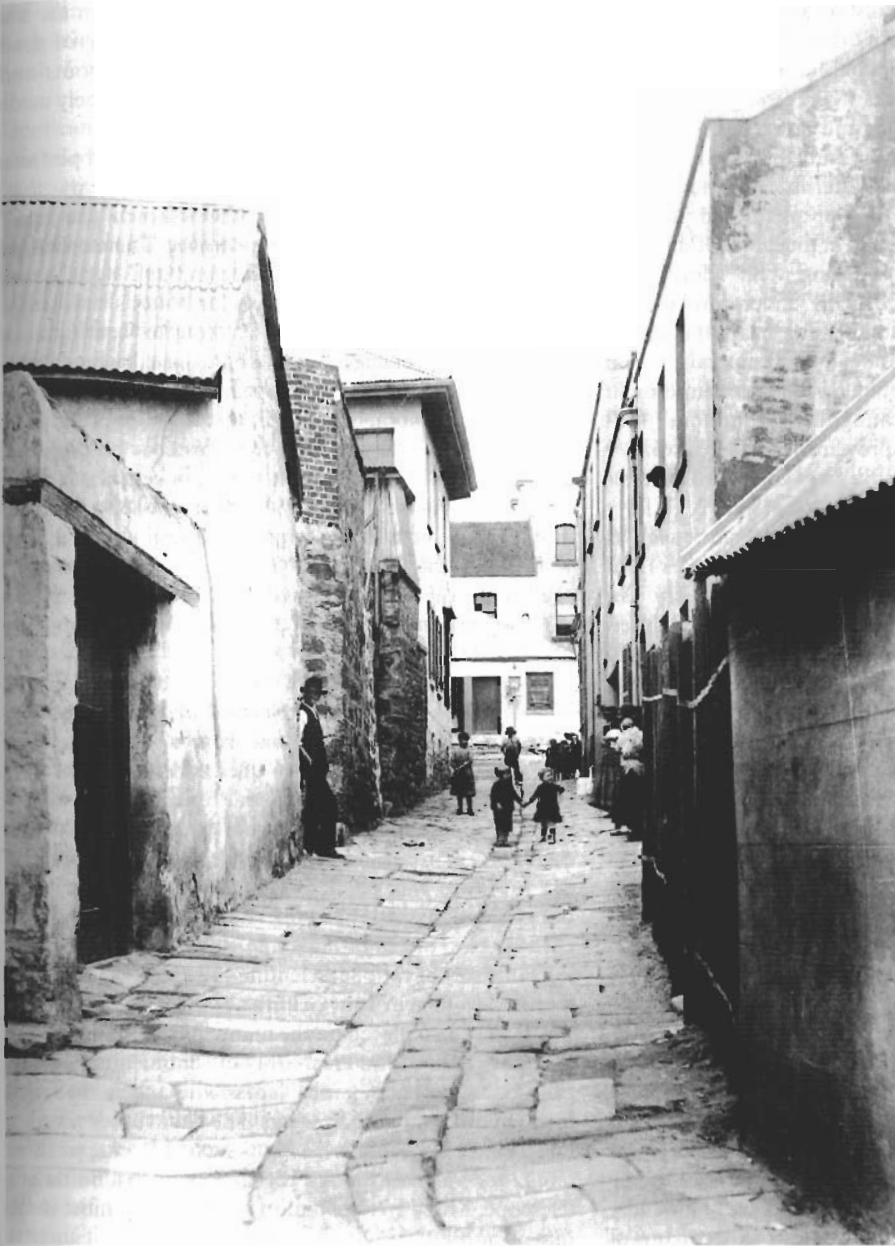
Fig. 6.3 Cribb's Lane, later called Cumberland Place, view to west, about 1900. This early lane bisected the site from east to west and by this stage was paved with sandstone blocks. On the left are gabled hotel stables, a walled yard and a substantial corner shop; on the right are an early house (c. 1810) and its yard, and a row of three flat-fronted terraces, with a corner hotel adjoining at the end. As in most of the photographs of this period, this one is constructed to suggest a 'crowded neighbourhood' scene, with local people carefully posed. The second woman on the right is hugging a large ceramic platter, typical of those found during the excavation.
