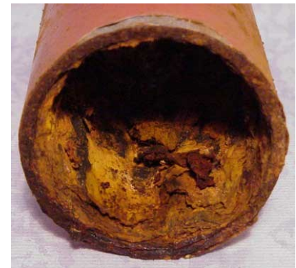
Rusty Pipe? CITY OF JGTON
