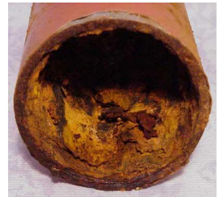
Rusty Pipe? CITY OF INGTON
