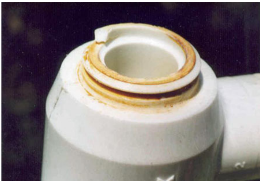
This polybutene pipe was damaged by a reaction between the plastic and chlorine in the water.
