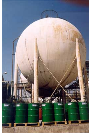
Figure 1. Propane Storage Tank
