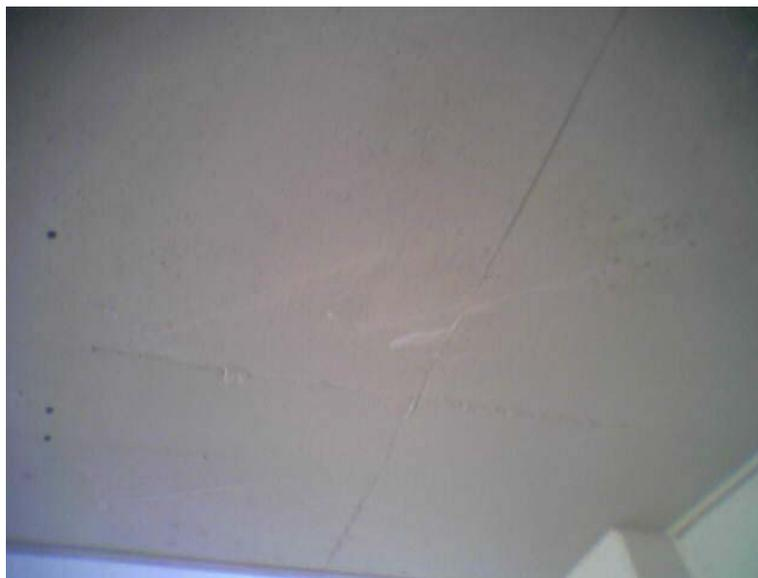
**Figure 3:** Cracks on the bottom of the same slab
