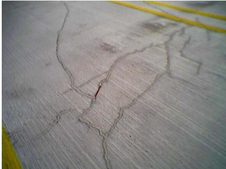
**Figure 2:** Cracks on the top floor of the parking structure
