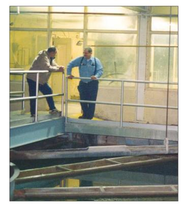
to 1,500–3,000 ntu within a few hours. The high turbidity levels could persist for up to 20 days before returning to normal levels. The high raw water turbidity would carry over through the clarifiers and filters, and we'd have periods when finished water turbidity approached or exceeded the 1.0 ntu maximum contaminant level (MCL).
