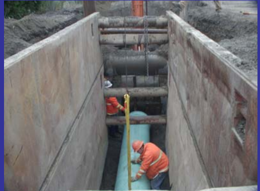
Gravity Sewer Installation
