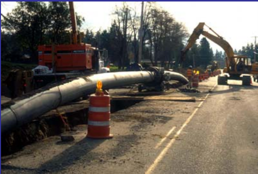
Force Main Installation
