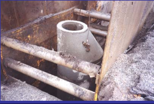
48-inch Concrete Sewer Manhole
