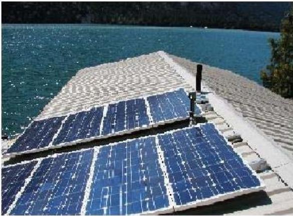
**Figure 31A:** The PV panels mounted on Visitors' Center roof before they were tilted to 34.6 degrees
