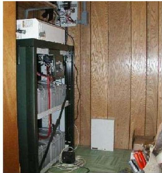
**Figure 31B:** The inverter/battery rack located in the Visitors' Center closet
