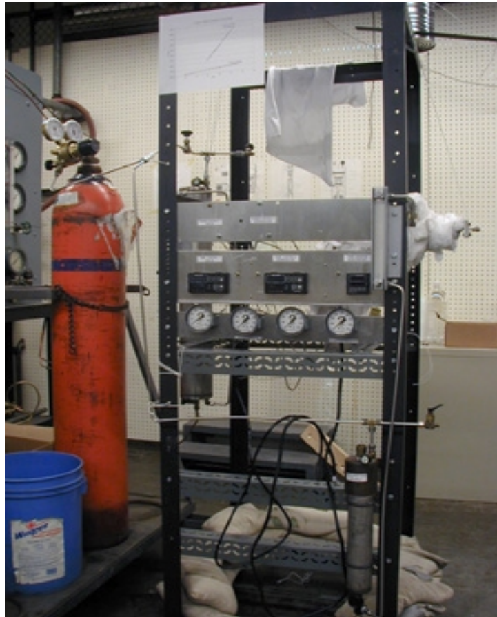
Figure 16: Front view of steam generator
