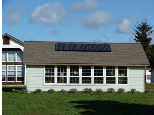
Figure 10. Completed installation of solar PV array.
