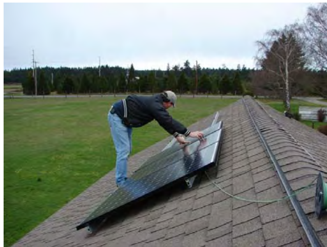
Figure 9. Installation of the five panel array.
