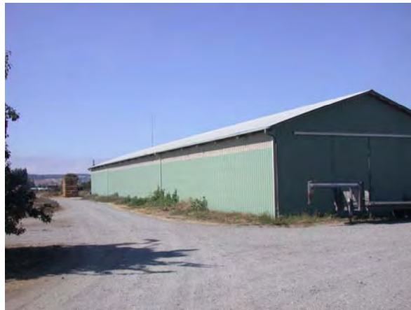
Figure 3. South facing roof on maintenance building at NPS farm #1
