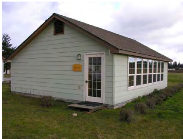
Figure 7. South facing roof on library at Au Sable Institute.
