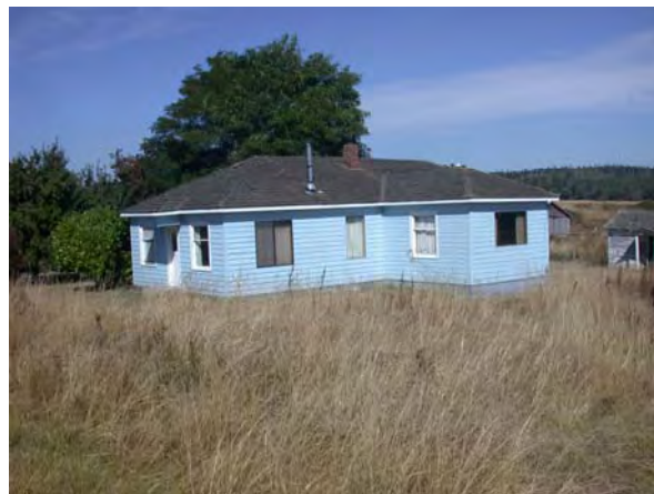
Figure 4. South facing roof on house at NPS farm #2.
