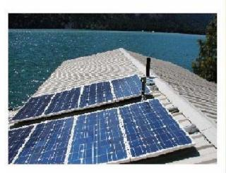
**Figure 31A:** The PV panels mounted on Visitors' Center roof before they were tilted to 34.6 degrees
