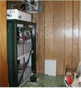
Figure 31B: The inverter/battery rack located in the Visitors' Center closet
