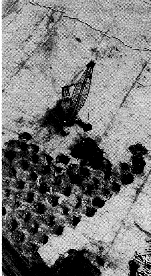
Figure 12.3 Aerial view of site undergoing soil improvement by dynamic compaction. The grid pattern on which the dynamic compaction weight is dropped, and the need for subsequent regrading and surface compaction, are evident from this photograph. (Photo courtesy of Hayward Baker).
