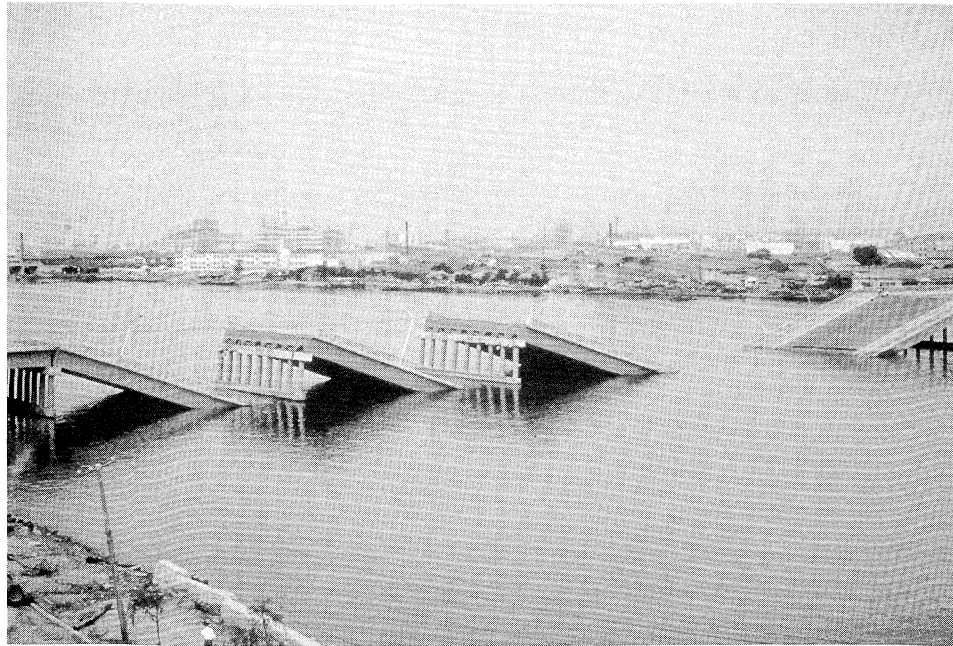
Figure 1.9 The Showa Bridge following the 1964 Niigata earthquake. Lateral spreading caused bridge pier foundations to move and rotate sufficiently for simply supported bridge spans to fall (courtesy of USGS).
