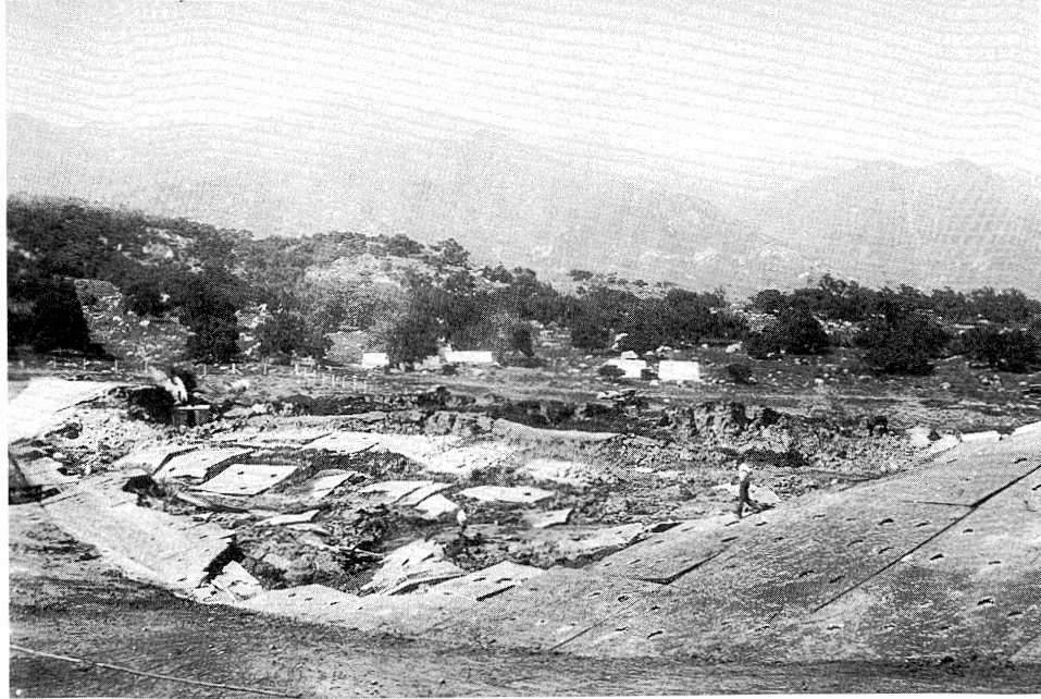
Figure 1.5 Liquefaction failure of Sheffield Dam following the 1925 Santa Barbara earthquake (K. Steinbrugge collection; courtesy of EERC, Univ. of California).
