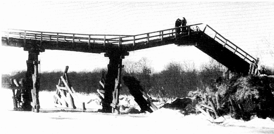
Figure 1.8 Effect of lateral spreading on a small bridge in Japan following the 1952 Tokachi-Oki earthquake. Lateral spreading of the soil at the abutment buckled the bridge deck (K. Steinbrugge collection; courtesy of EERC, Univ. of California).
