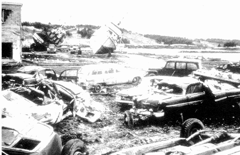
Figure 1.15 Tsunami damage in Kodiak, Alaska, following the 1964 Good Friday earthquake (courtesy of USGS).
