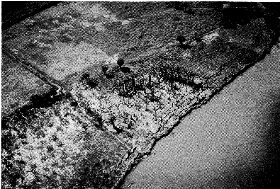
Figure 9.2 Lateral spreading of very flat ground toward the Motagua River following the 1976 Guatemala earthquake. Note orientation of ground surface cracks parallel to river bank (photo by G. Plafker; courtesy of USGS).
