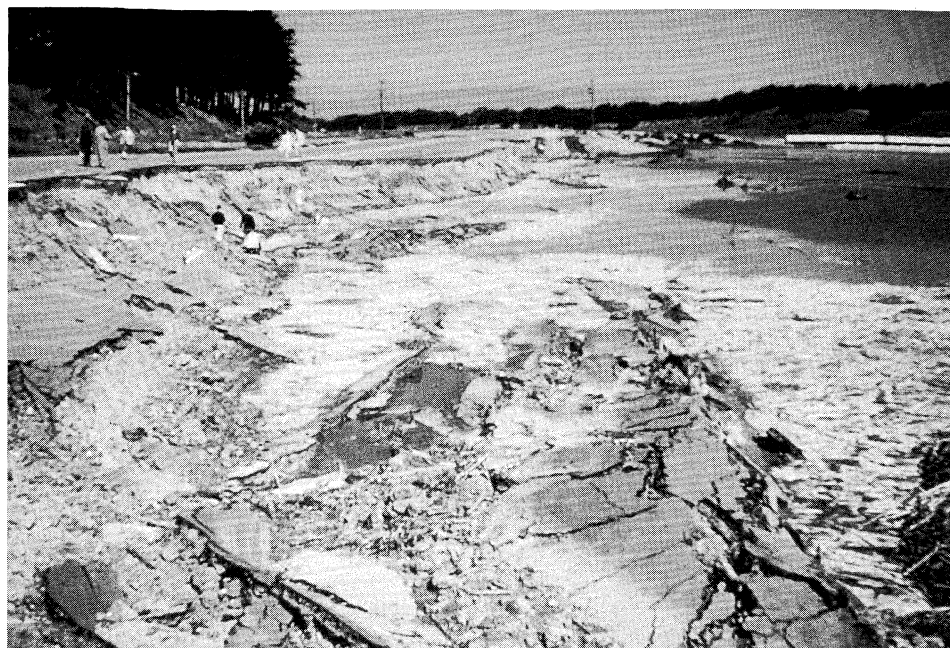
Figure 9.1 A small flow slide along the shore of Lake Merced in San Francisco in 1957 (photo by M. Bonilla; courtesy of USGS).
