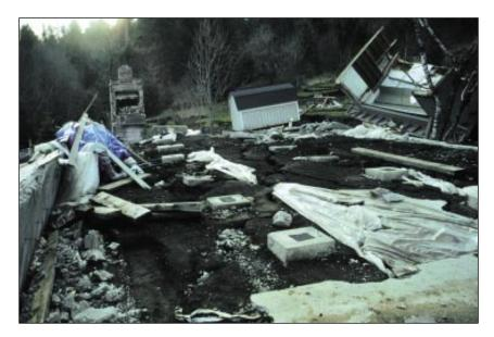
Figure 21. Effects of headscarp fractures on foundation of residence on Stevenson landslide.
