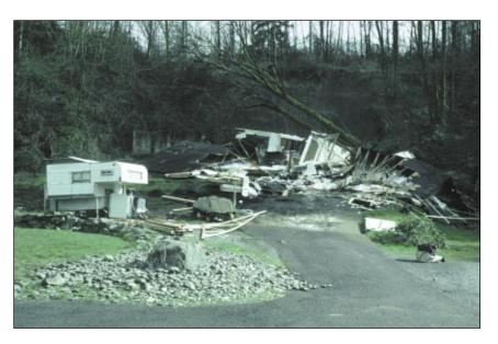
Figure 19. Small slump in northwest Vancouver that destroyed a residence located next to a steep slope bordering an old river terrace.
