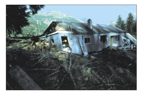
*Figure 15. House crumpled by block slide-debris flow shown in figure 16 near U.S.-12 east of Glenoma, Washington.*
