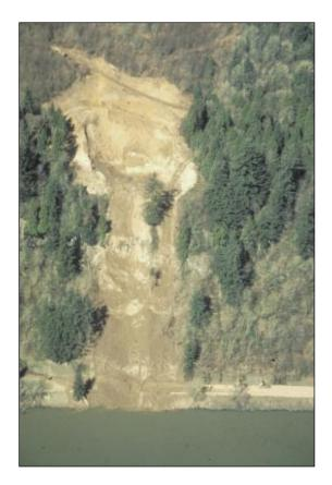
Figure 9. Large slumpdebris flow located about 5 mi west of Stella, Washington on SH–4.
