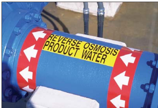
Reverse osmosis is highly effective for removal of most of these contaminants, but it is very costly, some of the water is lost as brine, and disposal of the brine is a significant problem.
