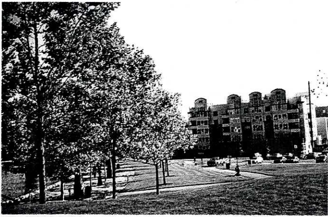
The park was a catalyst for residential development such as the McKee/Parkside on the south edge of the park. The five-story, wood-frame building above a podium garage is becoming the model for residential development in the area.
