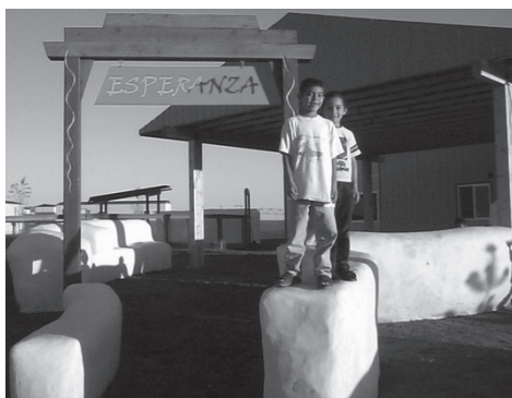
Figure 3. Strawbale wall at Esperanza Gathering Place, Mattawa, WA.
