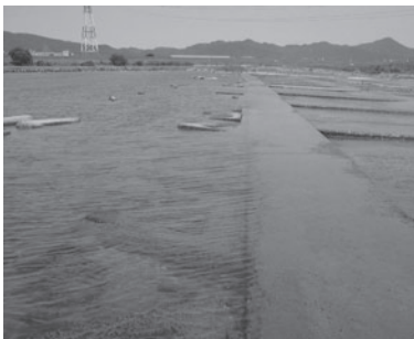
Figure 10. Walking path of the level concrete framework.
