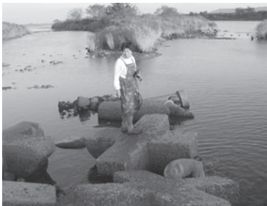
Figure 9. Stepping stones of concrete blocks.
