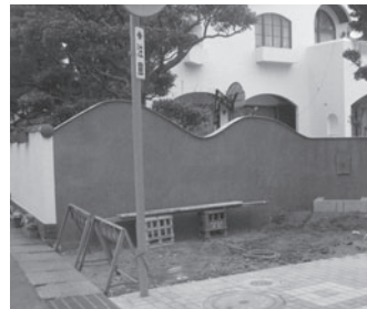
Figure 10. Construction of the Pocket Park.
