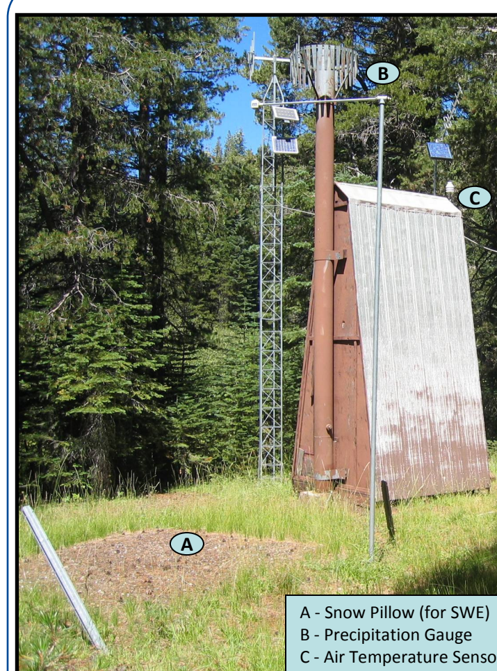
Example layout of a surface meteorological station with locations of measuring devices denoted by letter.
