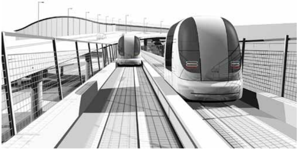
The ULTra podcar has been introduced at London Heathrow Airport.
