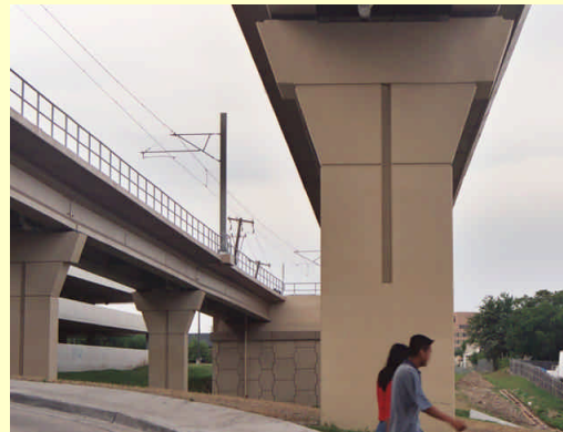
Massive support columns
