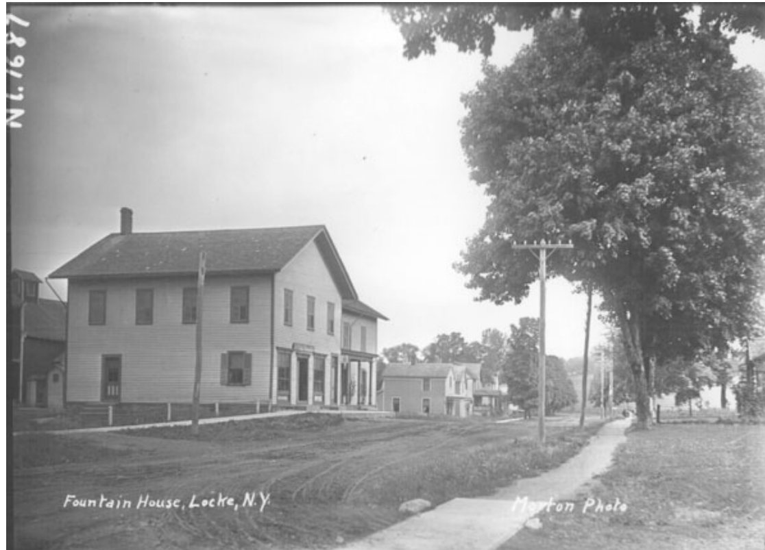
Muddy Main St. (Rt. 38) Locke, NY. c. 1907
