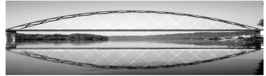
FIGURE 4-9B. A Compression Arch bridge completed in 2008 and known as the Blennerhassett Bridge crosses the Ohio River. The center span's length is 878 feet; the arch's rise is 175 feet; the roadbed's width is 107 feet. (Image manipulated to show lengthened arch)
