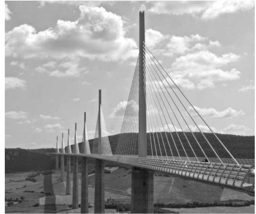
FIGURE 4-10. The Millau Viaduct, built in 2002-2004 for 394 million euros. The structure is 2,450 m long and supports a 32 m wide roadway which is at one point 270 m off the valley floor.
