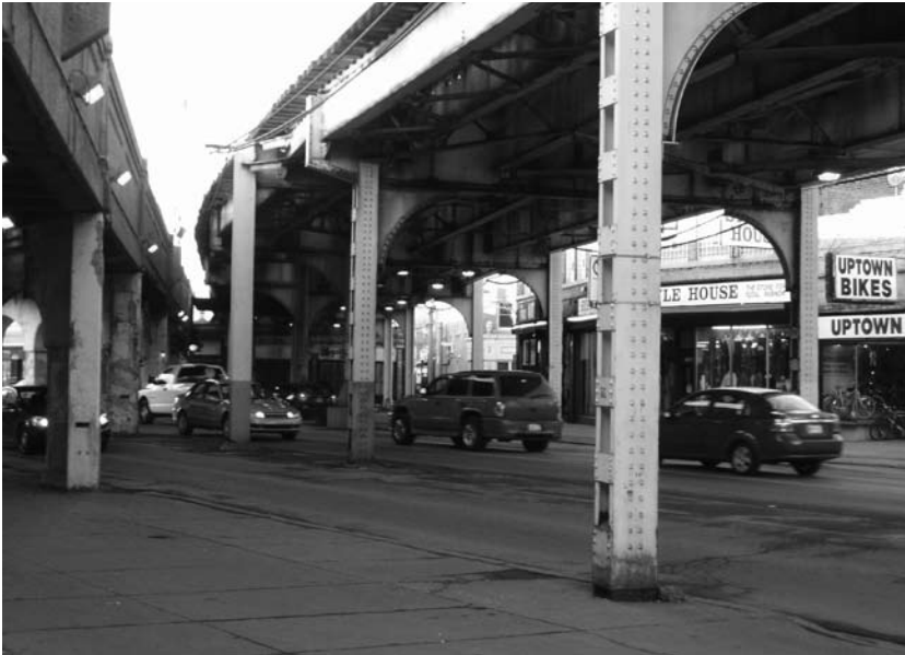
FIGURE 8-1 is a photograph of an elevated light rail system supporting full sized railroad cars of the famed Chicago "L" mass transit network.
