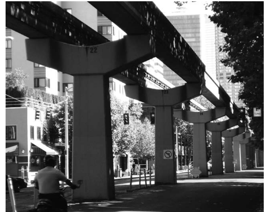
FIGURE 4-7. A concrete skeleton design is exemplified by a photograph of the monolithic, concrete, dual rail built for Seattle's World Fair monorail.
