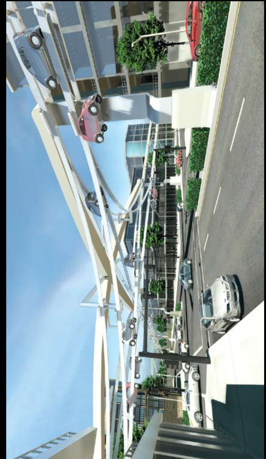
FIGURE 4-24b illustrates a full, high-capacity, 25 mph interchange above a common street intersection.
