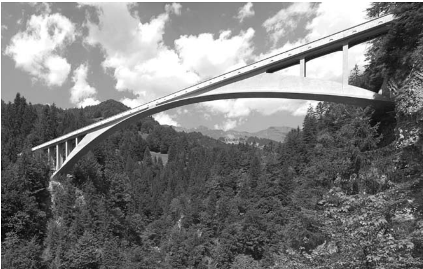
FIGURE 4-9A is a photograph illustrating the elegance that monolithic concrete structures can obtain. (source: http://fr.academic.ru/dic.nsf/frwiki/1441377 )
