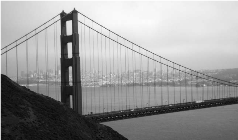
FIGURE 4–6A. San Francisco’s Golden Gate Bridge supports a roadway with the tensile strength of steel cables
