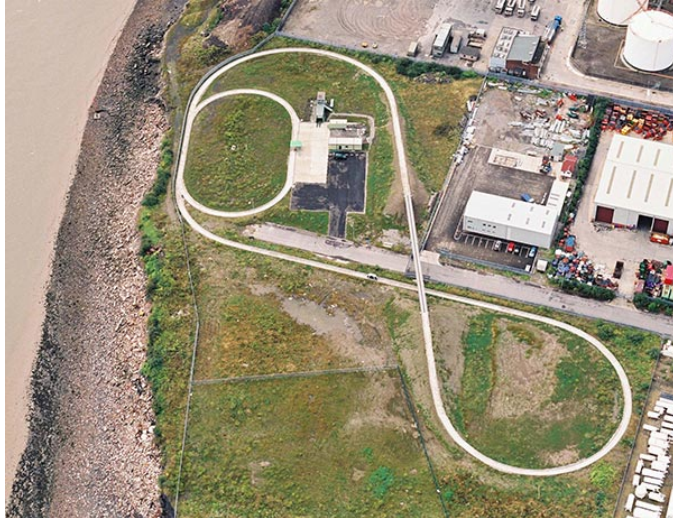
Aerial view of ATS test track
